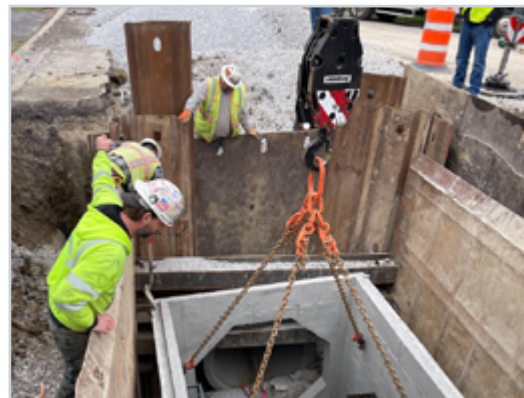
Baxter & Woodman performs construction observation services regularly.
