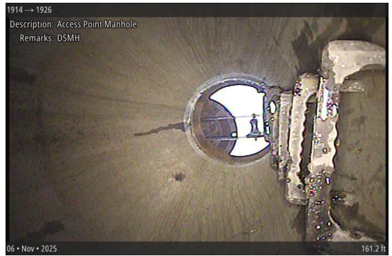
Access Point Manhole at 161.2 ft | DSMH
