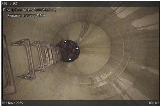
Access Point Manhole at 000.0 ft | starting USMH
