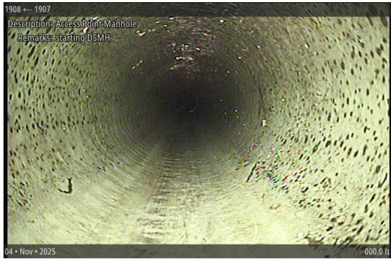
Access Point Manhole at 000.0 ft | starting DSMH
