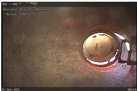
Access Point Manhole at 080.9 ft | DSMH
