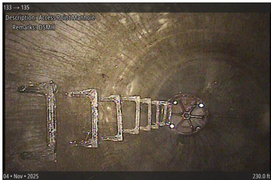
Access Point Manhole at 230.0 ft | DSMH
