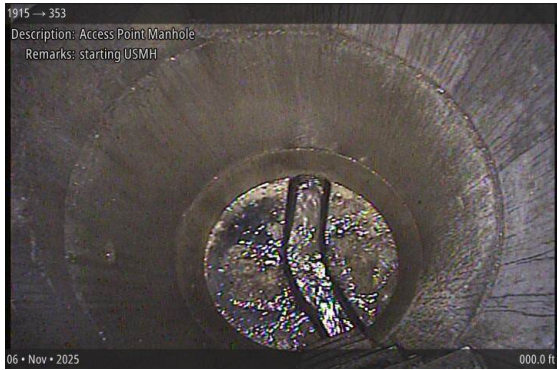
Access Point Manhole at 000.0 ft | starting USMH
