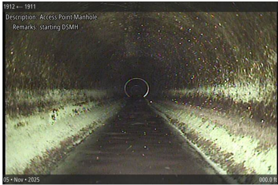
Access Point Manhole at 000.0 ft | starting DSMH
