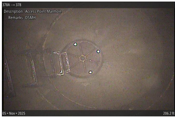
Access Point Manhole at 206.2 ft | DSMH
