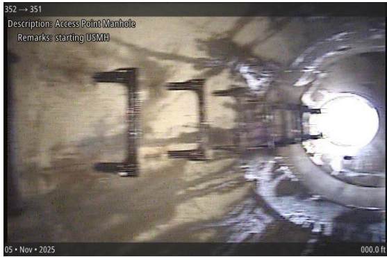
Access Point Manhole at 000.0 ft | starting USMH
