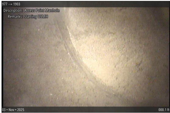
Access Point Manhole at 000.0 ft | starting USMH
