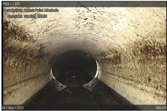
Access Point Manhole at 000.0 ft | starting DSMH
