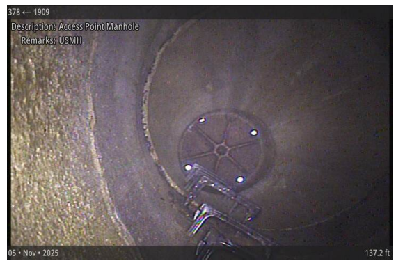
Access Point Manhole at 137.2 ft | USMH
