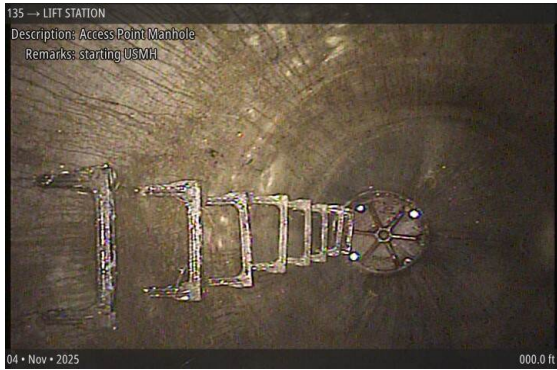
Access Point Manhole at 000.0 ft | starting USMH
