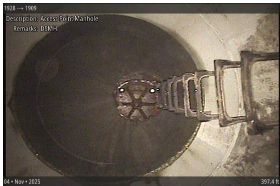
Access Point Manhole at 397.4 ft | DSMH
