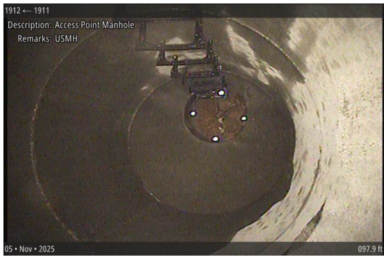
Access Point Manhole at 097.9 ft | USMH
