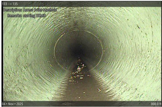
Access Point Manhole at 000.0 ft | starting USMH
