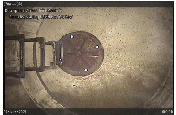
Access Point Manhole at 000.0 ft | starting USMH NOT ON MAP
