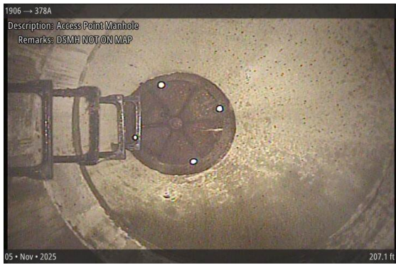
Access Point Manhole at 207.1 ft | DSMH NOT ON MAP
