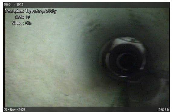
Tap Factory Activity at 296.4 ft, 10 o'clock
