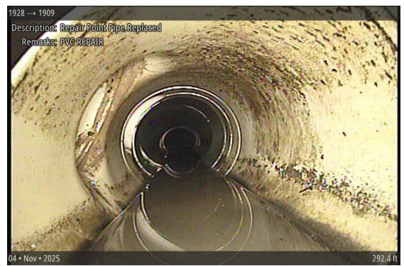
Repair Point Pipe Replaced at 292.4 ft | PVC REPAIR
