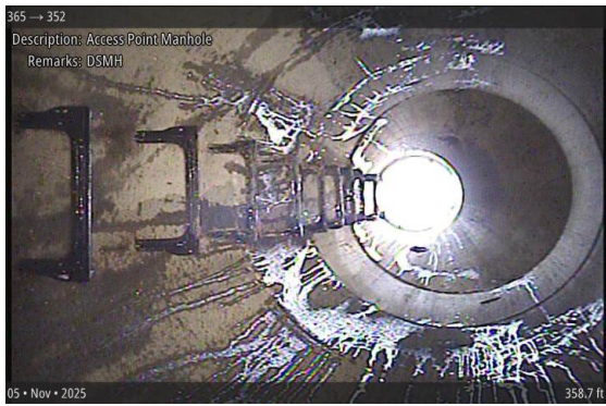
Access Point Manhole at 358.7 ft | DSMH
