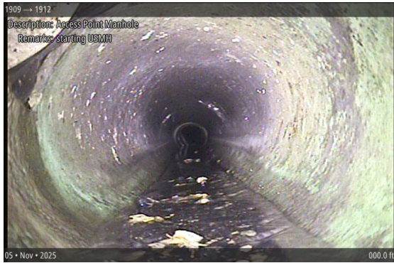
Access Point Manhole at 000.0 ft | starting USMH
