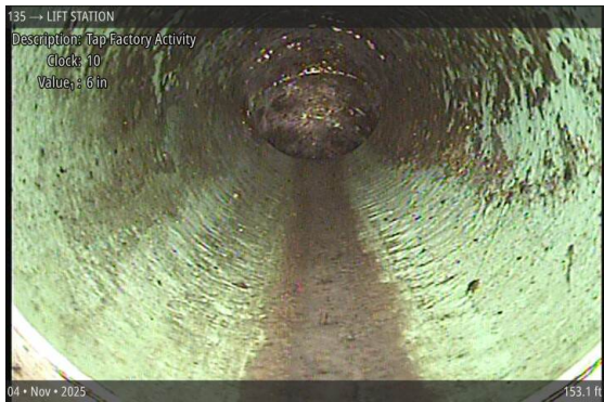
Tap Factory Activity at 153.1 ft, 10 o'clock
