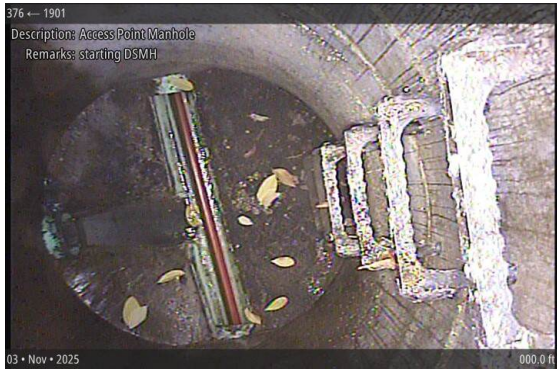
Access Point Manhole at 000.0 ft | starting DSMH
