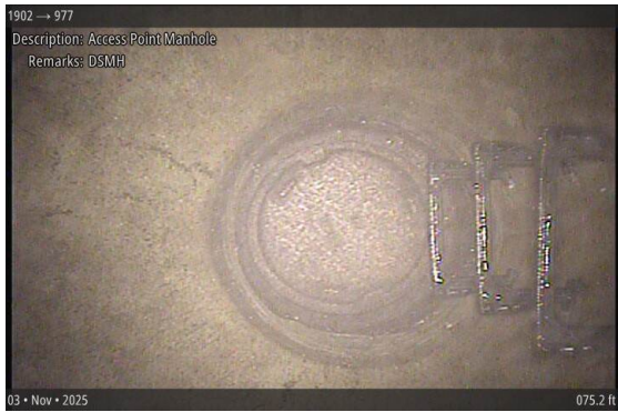
Access Point Manhole at 075.2 ft | DSMH
