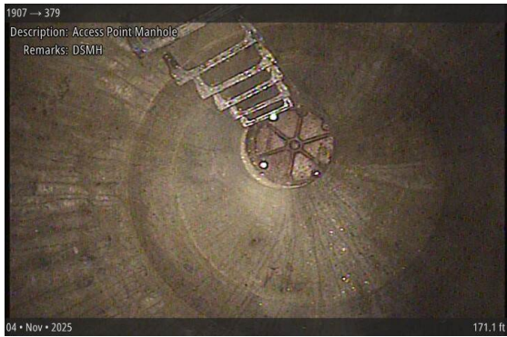
Access Point Manhole at 171.1 ft | DSMH
