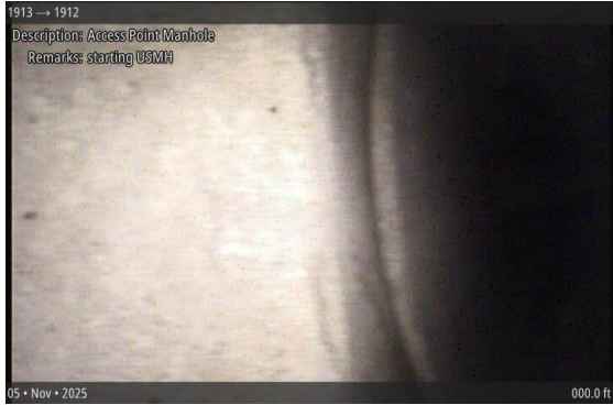
Access Point Manhole at 000.0 ft | starting USMH
