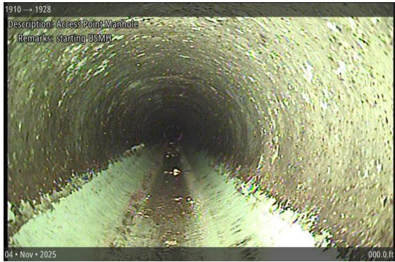
Access Point Manhole at 000.0 ft | starting USMH
