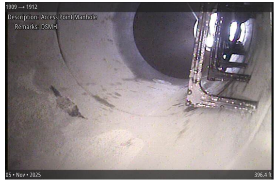
Access Point Manhole at 396.4 ft | DSMH
