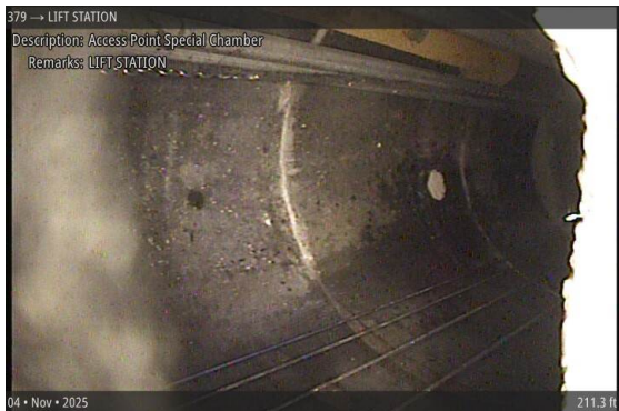
Access Point Special Chamber at 211.3 ft | LIFT STATION
