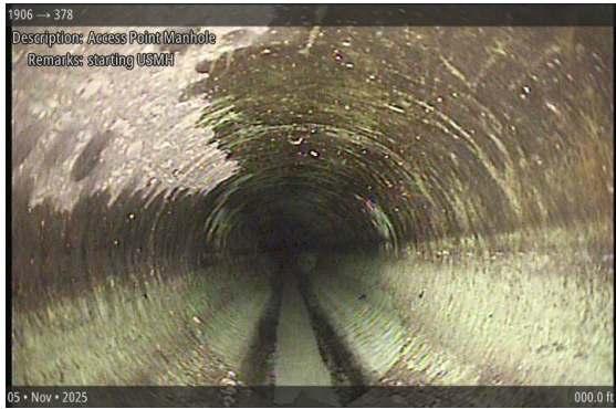
Access Point Manhole at 000.0 ft | starting USMH
