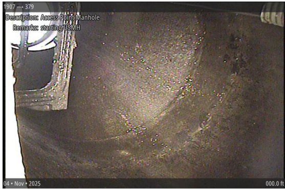
Access Point Manhole at 000.0 ft | starting USMH
