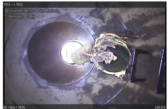
Access Point Manhole at 250.8 ft | DSMH
