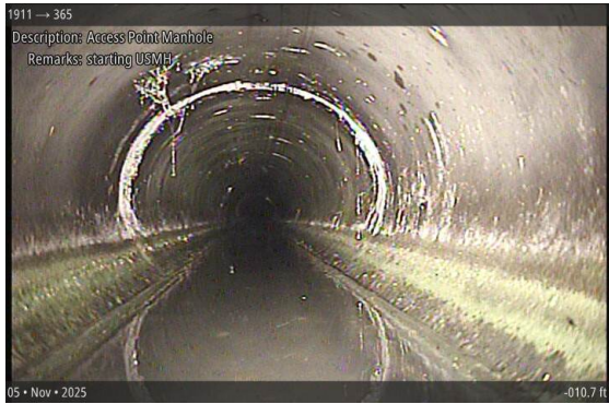
Access Point Manhole at 000.0 ft | starting USMH
