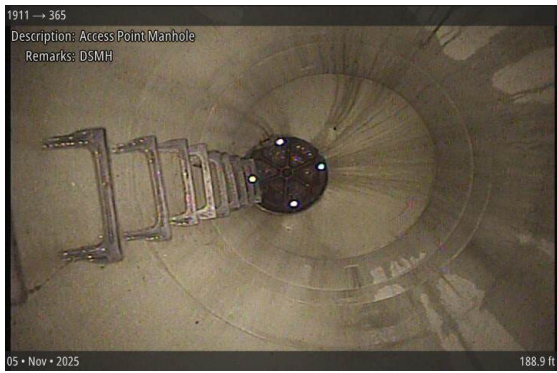
Access Point Manhole at 188.9 ft | DSMH
