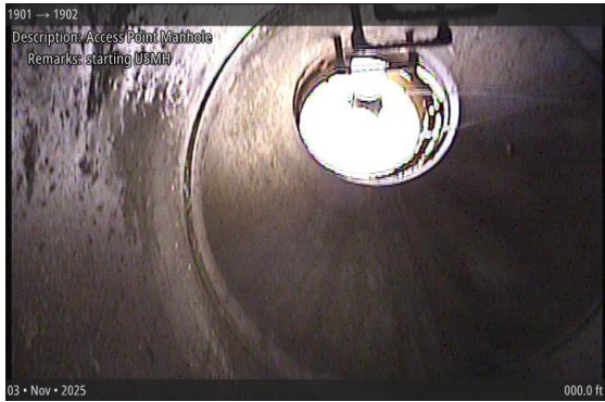
Access Point Manhole at 000.0 ft | starting USMH
