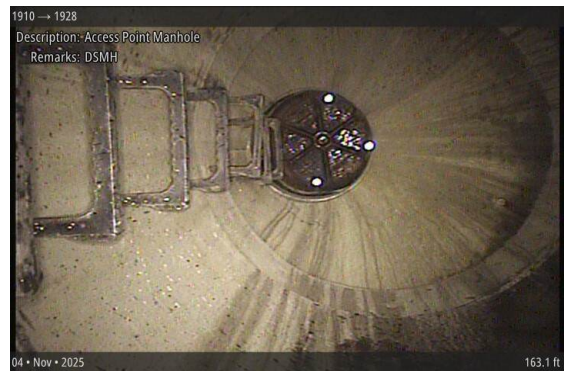
Access Point Manhole at 163.1 ft | DSMH
