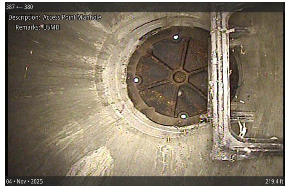
Access Point Manhole at 219.4 ft | USMH
