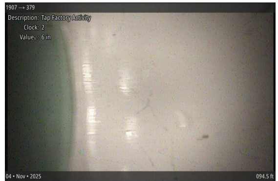
Tap Factory Activity at 094.5 ft, 2 o'clock
