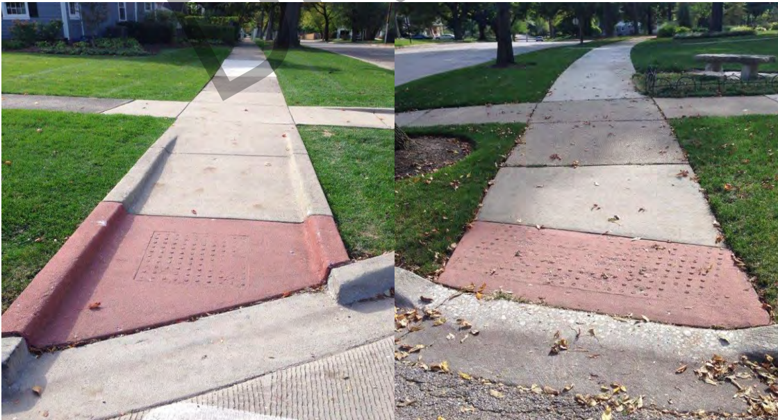
The above crosswalks were installed to meet the previous ADA standards. They are non-compliant in the current ADA standards and make up the majority of the non-compliant intersections in the Village.
