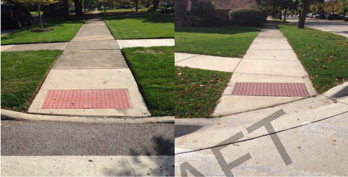
The above crosswalks are compliant with the current ADA standards. All future construction will include the installation of similar crosswalks.
