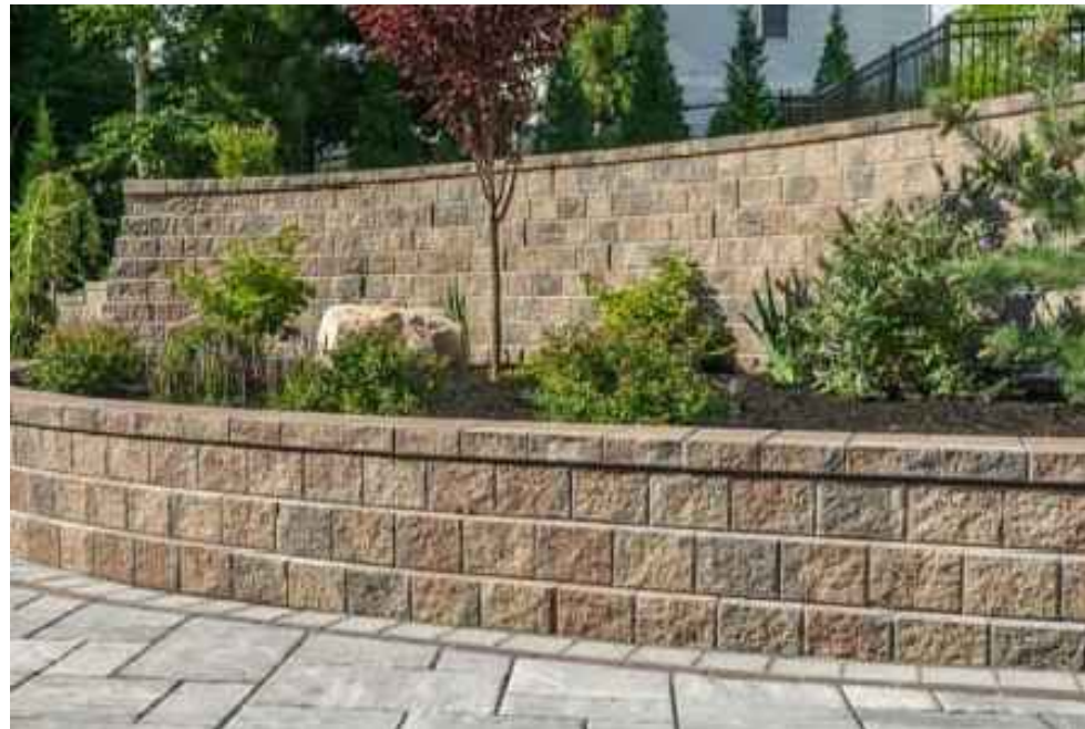
4 - Concord Retaining Wall
