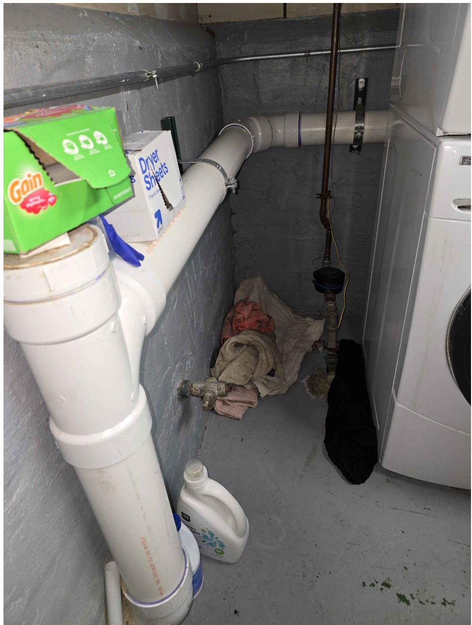
3 METER LOCATION: BASEMENT SERVICE PENETRATION INSIDE HOUSE: FLOOR SCALE: NTS
