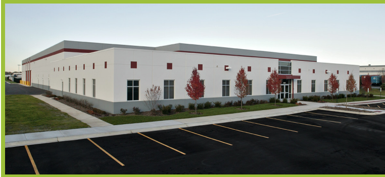
Village of New Lenox - Public Works Facility
