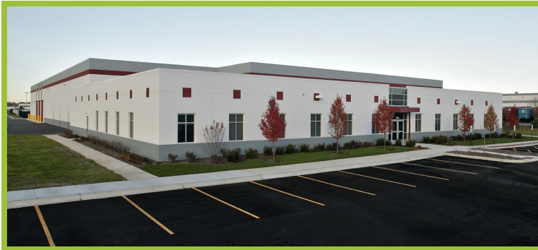
Village of New Lenox - Public Works Facility
