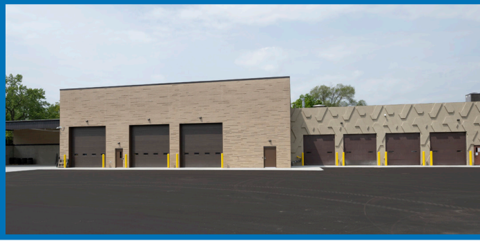
Village of Lombard - Public Works - Public Works Garage Addition
