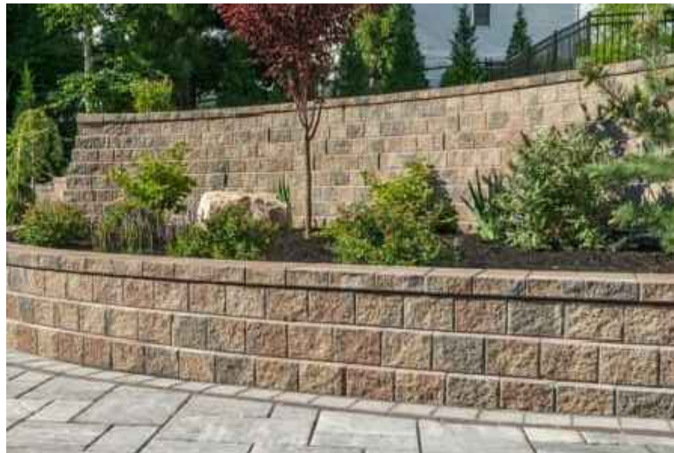
4 - Concord Retaining Wall
